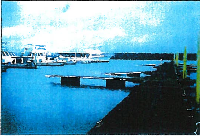
Main Gang Way & Finger Slips
