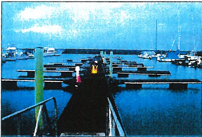
Main Gang Way & Finger Slips
