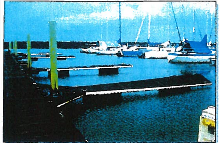
Finger Slips, pontoons & Steel Piles
