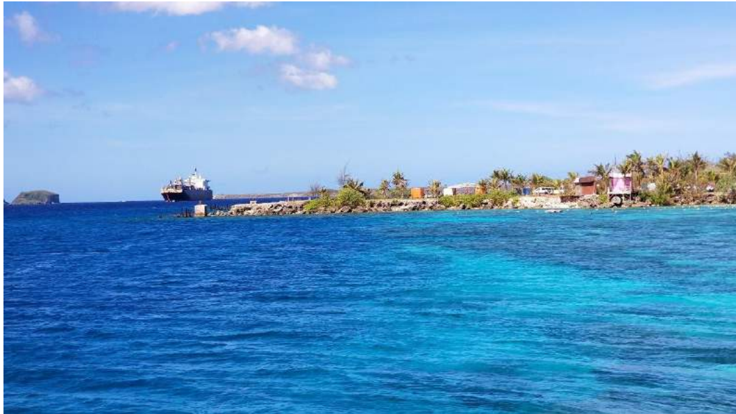
Photo 1. East pier of Dog Leg Pier, facing west, March 2019.
