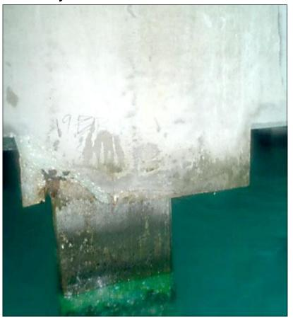
Pilecap 19B – Progressed damage: spalling and exposed rebar
