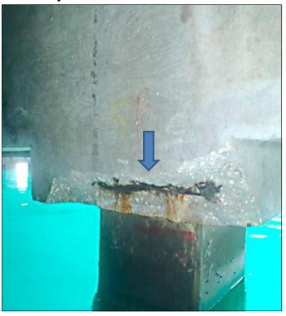
Pilecap 15B – Progressed damage: spalling and exposed rebar
