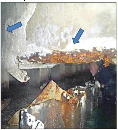
**Bent 9D-E – Progressed damage: spalling**
